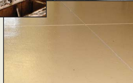
Epoxy floor preparation and surface etcher.
